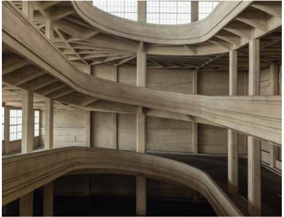
Lingotto, helix access ramp
