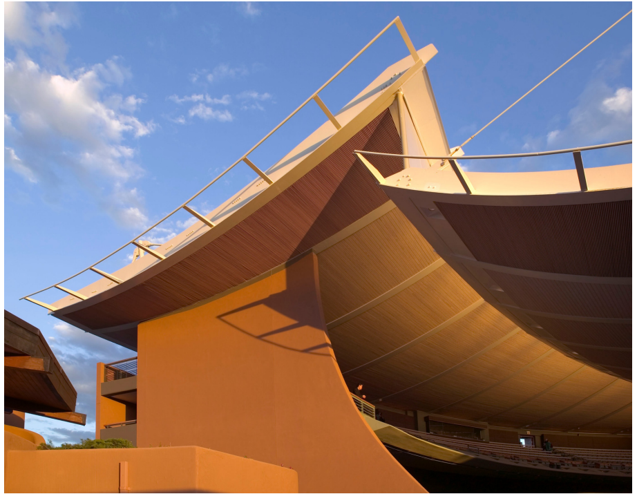
Santa Fe Opera theatre, photo courtesy of Santa Fe Opera.
